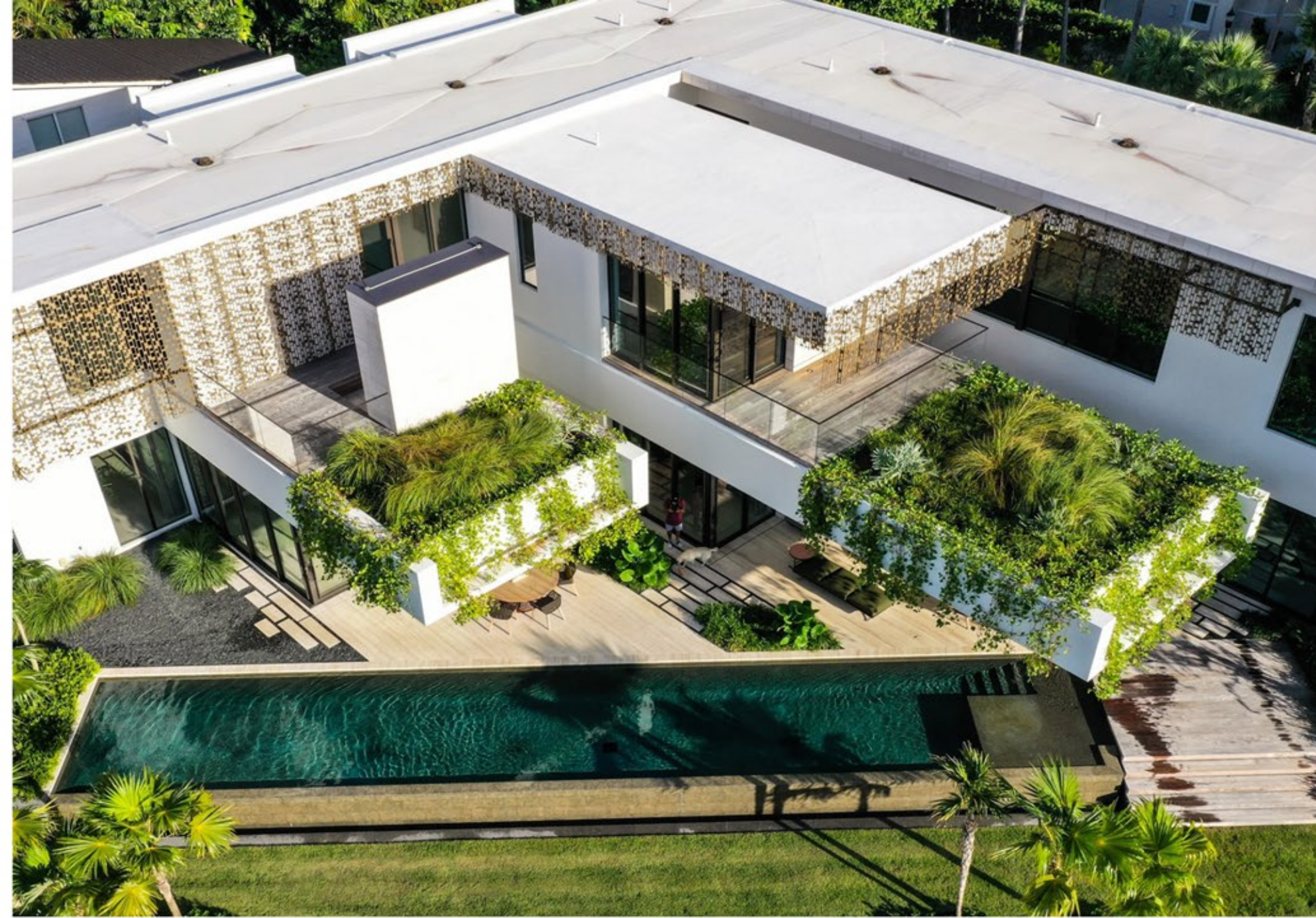
Private Residence Defined by a sequence of outdoor rooms, the garden harmoniously unifies the architecture with its surrounding environment.
