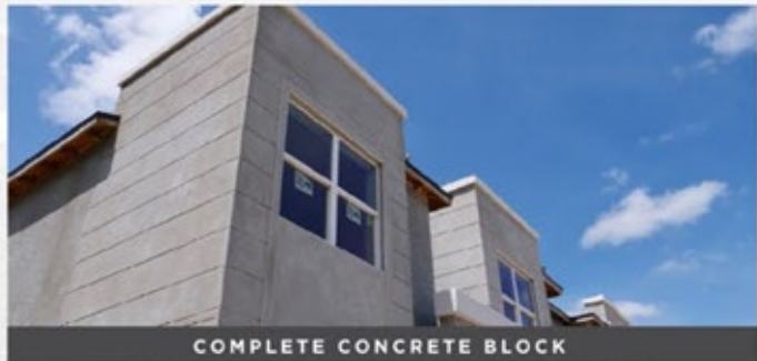
COMPLETE CONCRETE BLOCK
